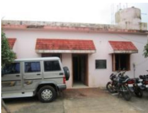
EOC constructed under DRM programme (2006), used for other official purpose
