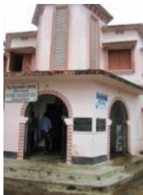
EOC constructed by District Administration (2003), now used for Emergency Operation Centre
