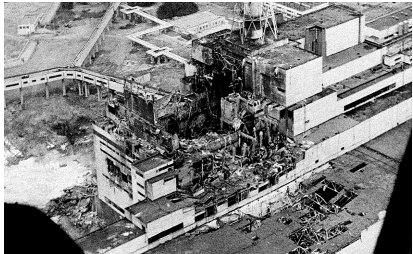
Fig3: Damaged Reactor 4 facility
